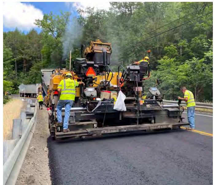
Wilmington-Brattleboro NH 2971(1) Paving Operation
