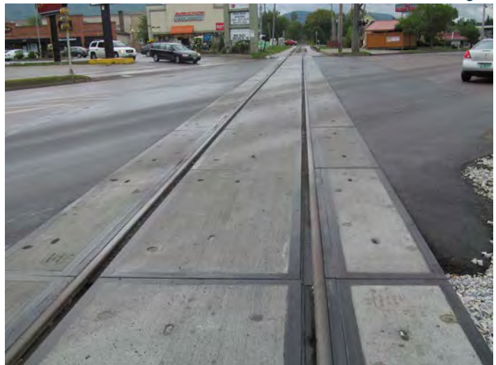
AFTER: Rutland South Main Street Grade Crossing
