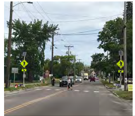
Pine Street in Burlington, VT – Rectangular Rapid Flashing Beacons (RRFB)
